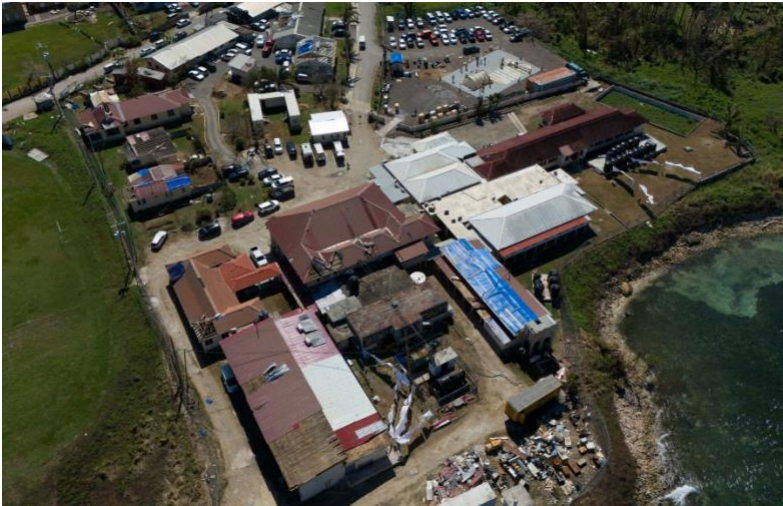
Project HOPE constructs a field hospital near the parking lot of Noel Holmes General Hospital in Lucea, Jamaica, which sustained significant damage and has tarps covering roofs. Photo by Charlie Cordero for Project HOPE, 2025.
